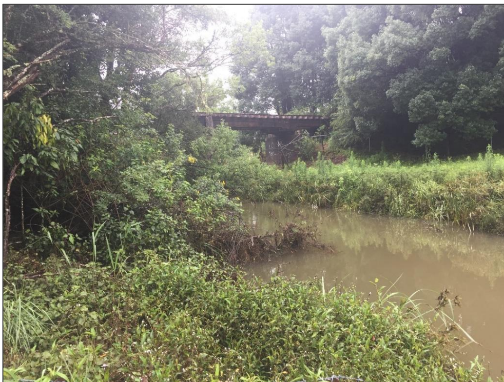
Figure 1-3 Railway Bridge over Maori Creek
