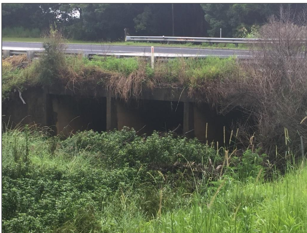
Figure 1-4 Culverts structures under Lismore Road on Maori Creek
